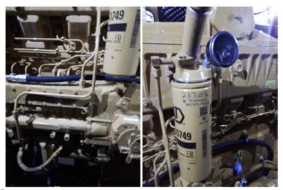
4. Fuel lines and piping - the supply and return piping needs to be replaced.
